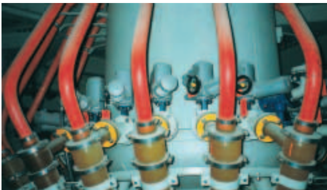
AUMA part-turn actuators in the desulphurisation unit of a power plant.
