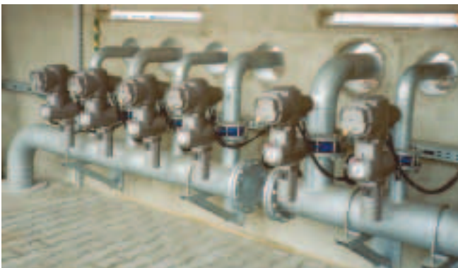
AUMA part-turn actuators with AUMA MATIC integral controls in a tank farm in Poland.
